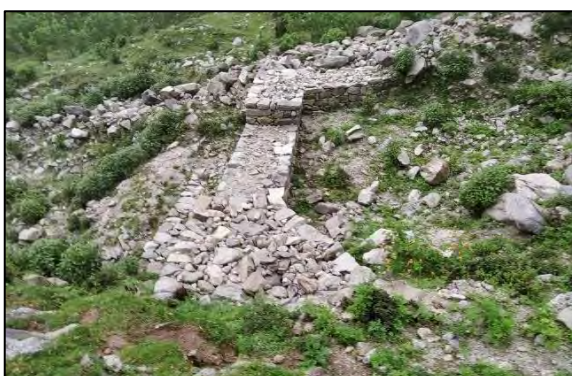
Check Dam, Rajaein VFMS
